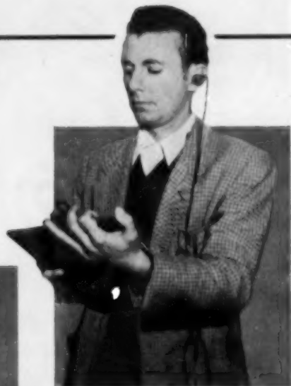
The "Conelrad" receiver in operation. A hearing-aid type earpiece and small plastic box comprise the entire receiver.
