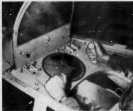
Mockup of cockpit showing position of the two TV screens. One plate is mounted vertically while a second lies horizontally between pilot's hands.
